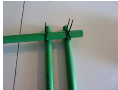
Figure 2. In this picture we can see how we can keep on fastening pipes together in order to construct the frame of the platform.
